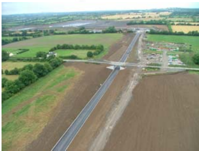
Knockharley Landfill - Roadworks
