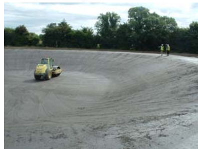
Knockharley – Clay / HDPE liner
