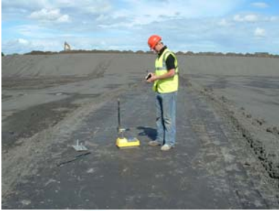
Liner CQA – NDM testing
