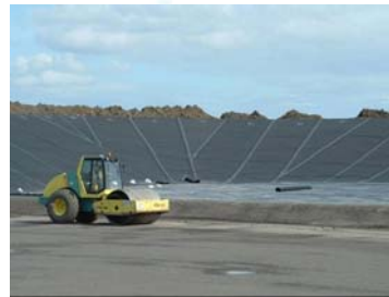
Knockharley – Clay / HDPE liner
