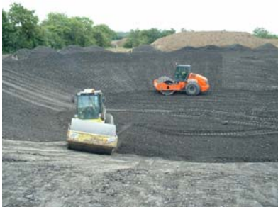
Knockharley – Clay / HDPE liner
