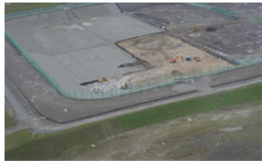
Controlled landfilling into lined cells
