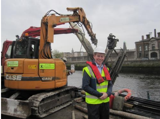
Photo: Robert on site on Wolfe Tone Quay, Dublin
