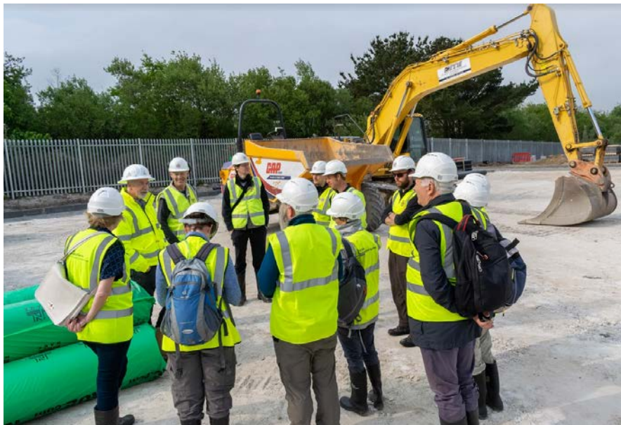
Figure 12: Visiting the United Downs geothermal project site in Cornwall.
